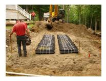
Eljen has developed improved water management on slopes. This system encourages recycling of pretreated effluent. It minimizes the footprint and eases access and installation in difficult-to-reach locations. Eljen
