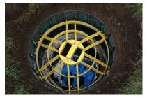
installation of septic tanks for many installers. The Equalizer is used to self-regulate the flow of effluent to the leach field.
