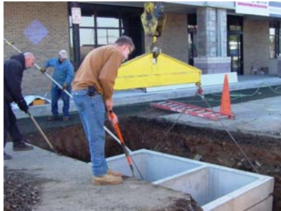
Installation at Southbury Plaza
